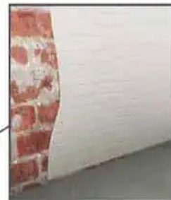
4. Apply Scratch Coat Apply a rough coat of at least 5mm thick. This will act as an anchoring layer.
