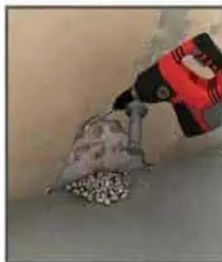
1. Prepare the Wall Remove damp/salt contaminated plaster.
