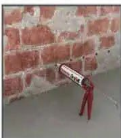
2. Drill Holes 12mm holes drilled at regular intervals into mortar bed
