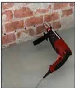
2. Drill Holes 12mm holes drilled at regular intervals into mortar bed
