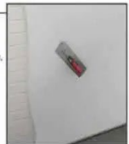
5. Apply Plaster Coat Once scratch coat has become firm, apply the plaster again with at least 15mm-20mm thick.
